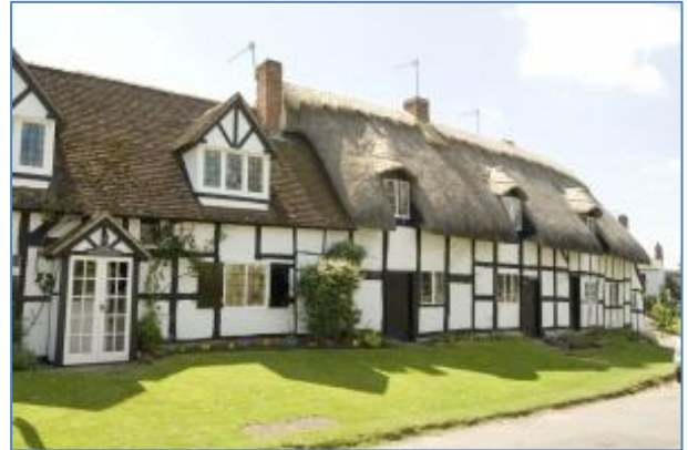
Figure 4 - Church Street (in the Conservation Area)
